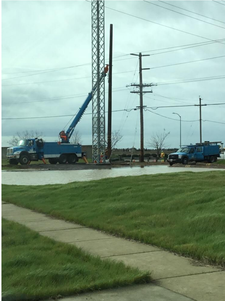
Photo 1: CPUC EM observed crews removing a guard structure at structure 0/10.
