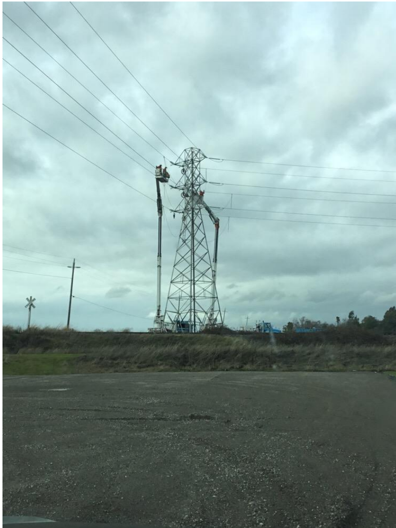
Photo 2: Crews were observed installing insulators at structure 1/13.
