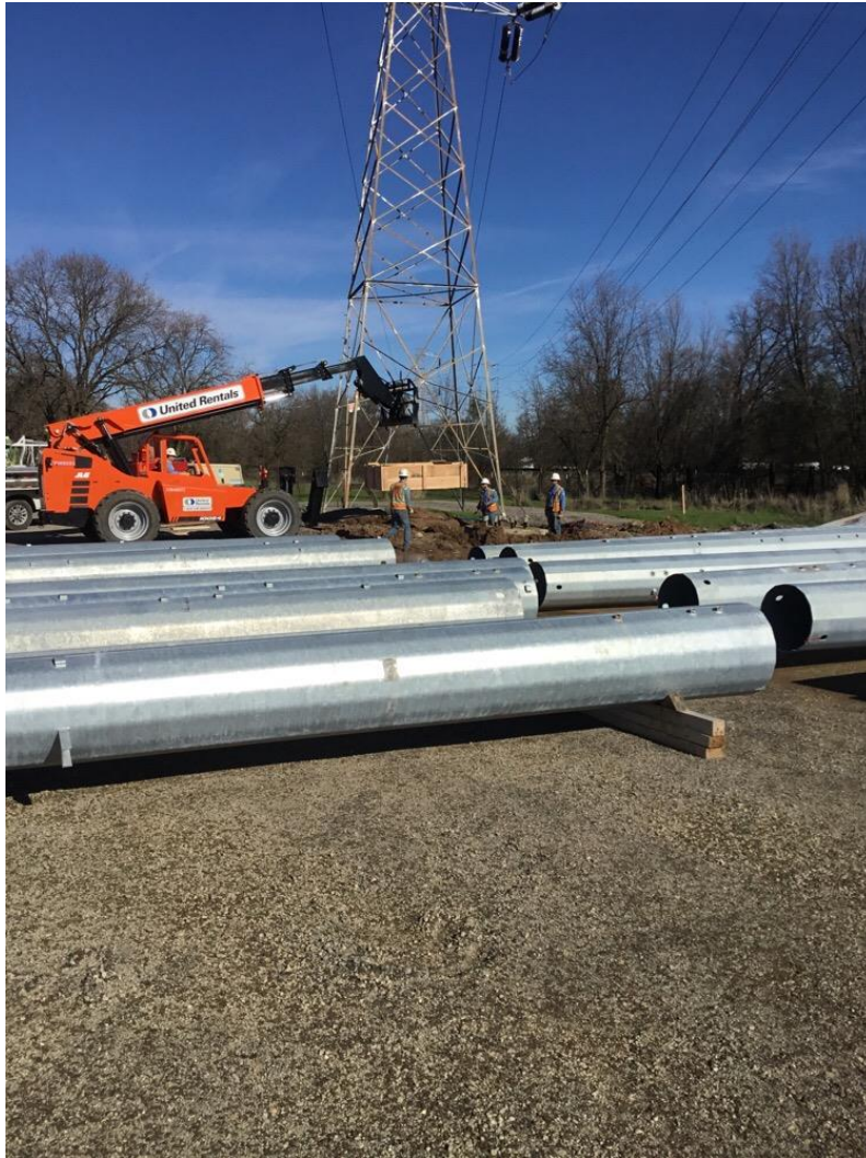
Photo 4: Crews were observed installing framing for pouring foundation at structure 4/31.
