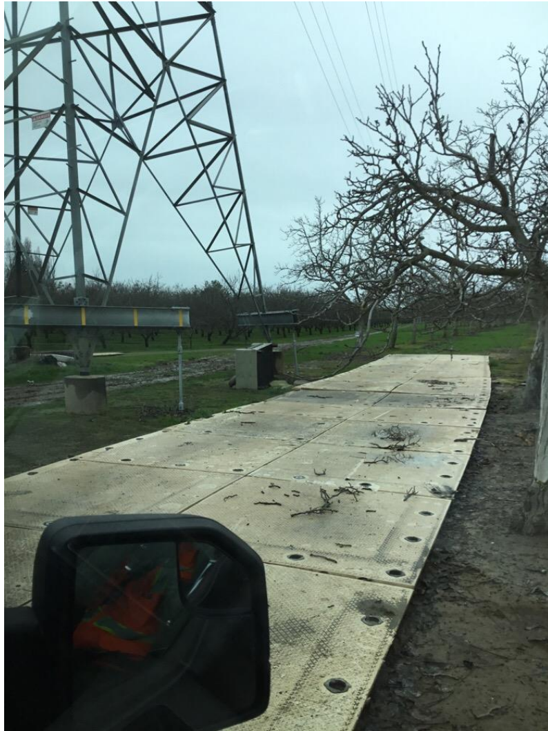
Photo 3: Track-out mats were installed at structure 3/31 to prevent track-out.
